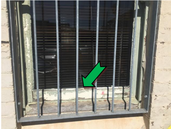
Photo 1. Exterior, ground level, throughout window frames – non asbestos-containing external window caulking.
